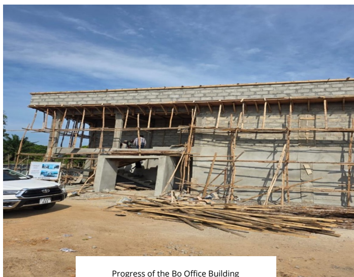
Progress of the Bo Office Building
